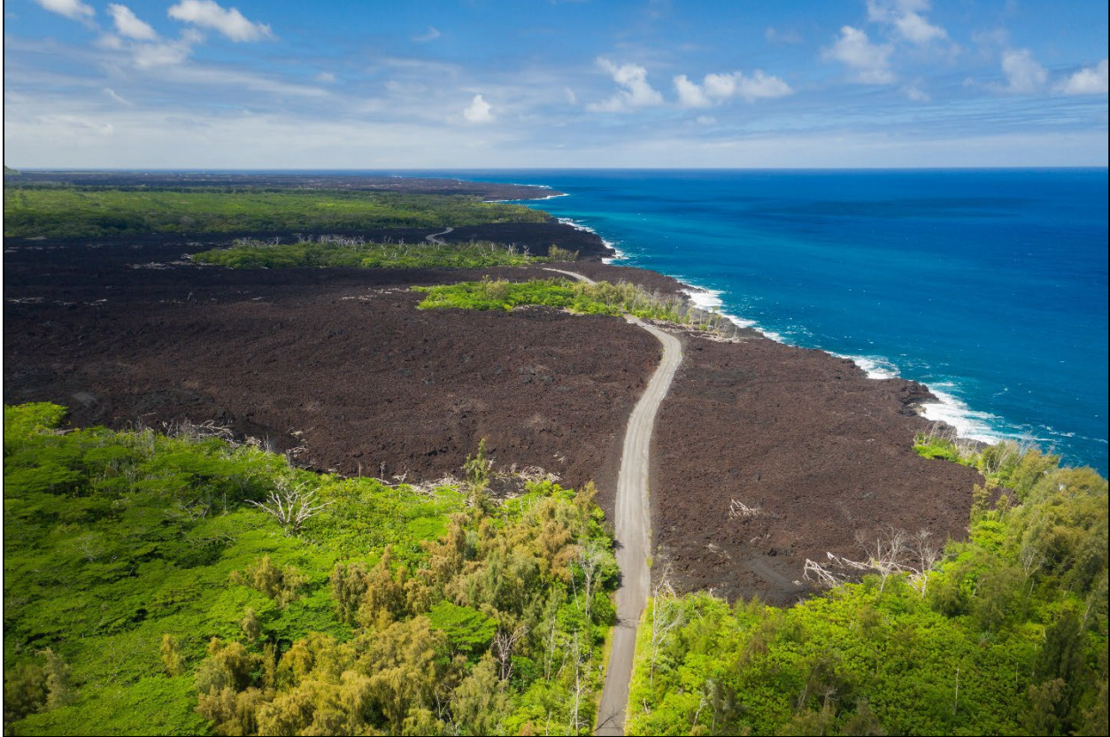
Photo 4. Hardened lava across Highway 137 near MacKenzie State Recreation Area, facing northeast (photo shows temporary road rebuilt after 2018 lava flow)
