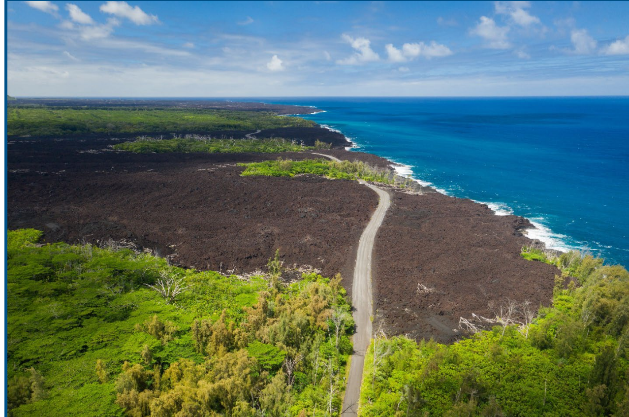
Photo of hardened lava across Highway 137 near MacKenzie State Recreation Area, facing northeast (photo shows temporary road rebuilt after 2018 lava flow).
